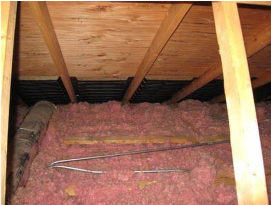
(left) Attic space after air chute installation.
