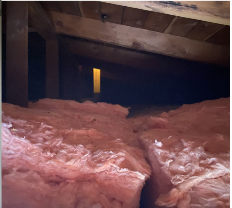
(left and below) Currently has non-breathable soffit 2nd floor and no air chutes in attic space
