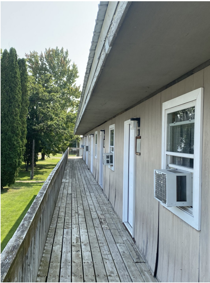
(left and below) Currently has non-breathable soffit 2nd floor and no air chutes in attic space
