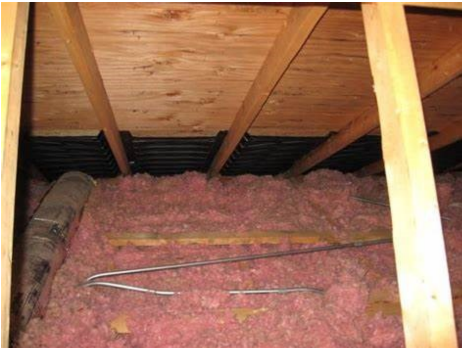
(left) Attic space after air chute installation.
